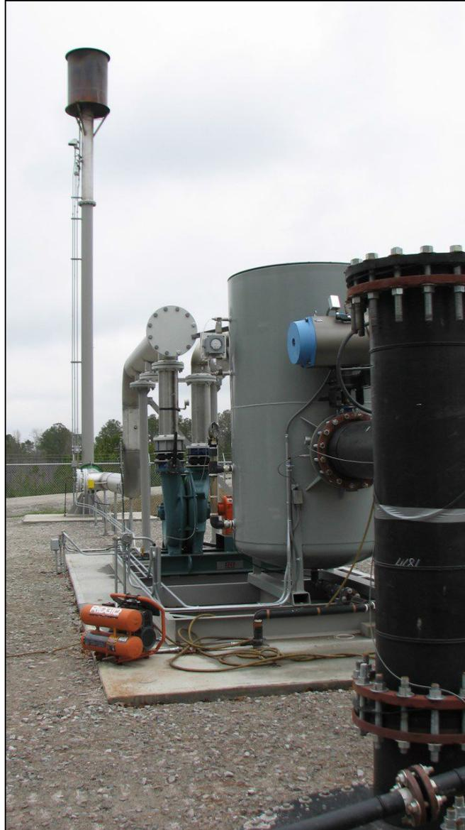
This methane extraction and condensate removal system consisted of a 60 HP gas extraction blower and 3500 SCFM candlestick flare that was designed and manufactured by PRM. Includes a full SCADA control panel package with integrated PLC. The system provides gas to a 6MW generator plant using 24 packages engines. PRM provided system manufacturing, integration, installation, and startup. In 2017 the system was upgraded to include two more 60HP blowers to increase production for the client.
