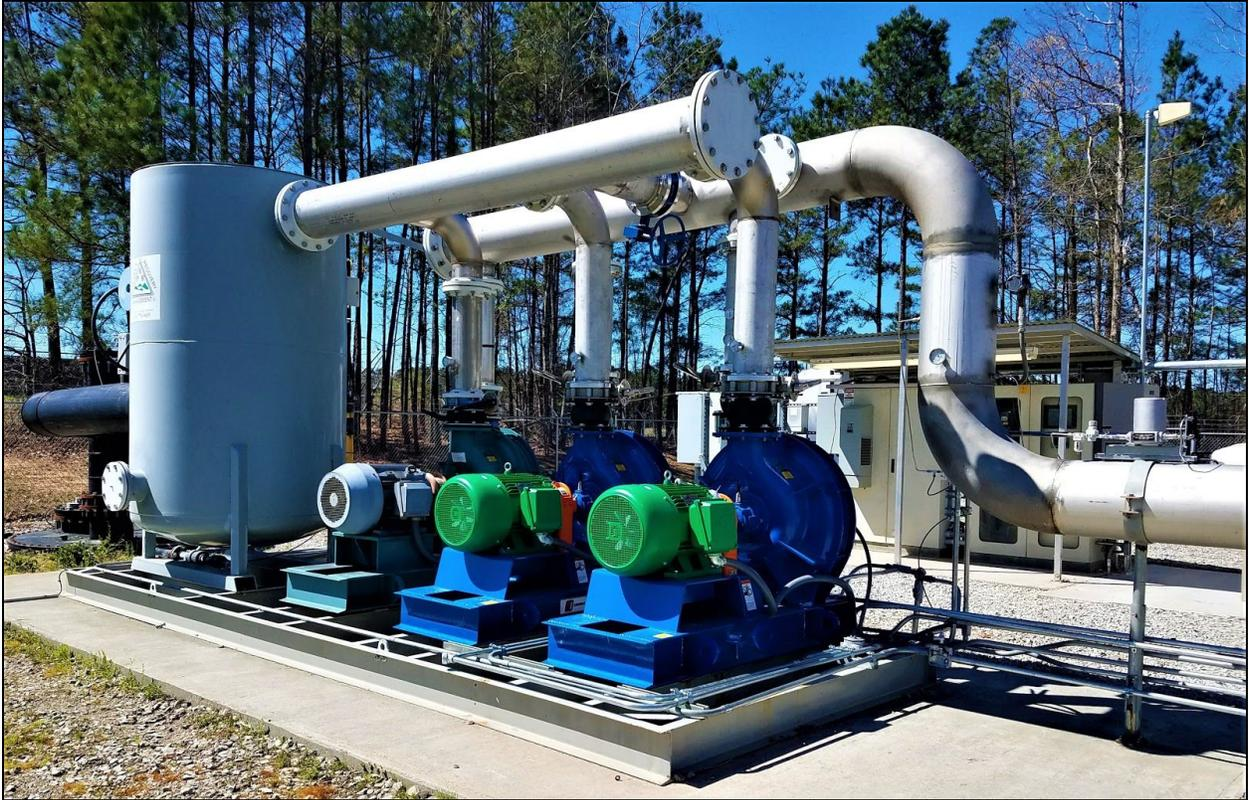
Prm provided a landfill extraction blower system upgrade per Clients RFQ and project manual. Two additional LFG blowers were added to the existing skid unit onsite. PRM provided Variable Frequency Drives (VFD) for each new blower motor along with a new control panel for complete system operations.
