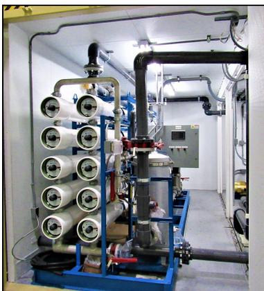
PRM provided a fully integrated and packaged Reverse Osmosis Treatment system. The dual side-by-side Connex container system included Tandem 8'x20' HC Single Trip containers modified to allow for a single 16'x20 site structure for housing the equipment, 2 AMT Model 315B-98 SS pumps, 480V 3phase 3HP TEFC Motors for premium efficiency, VFD controls with PID loop from a Pressure transmitter, and a 24,000Btu HVAC Minisplit system for interior heating and cooling/dehumidification.
