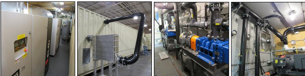
This SVE/AS system was housed in two 8' x 40' Connex containers. One enclosure housed the SVE systems and three Rotary claw compressors. This enclosure was rated for a Class I Div 2 location. The second enclosure housed two Rotary screw compressors and air dryers. This enclosure included a closed off room that contained the main breaker panel and controls.
