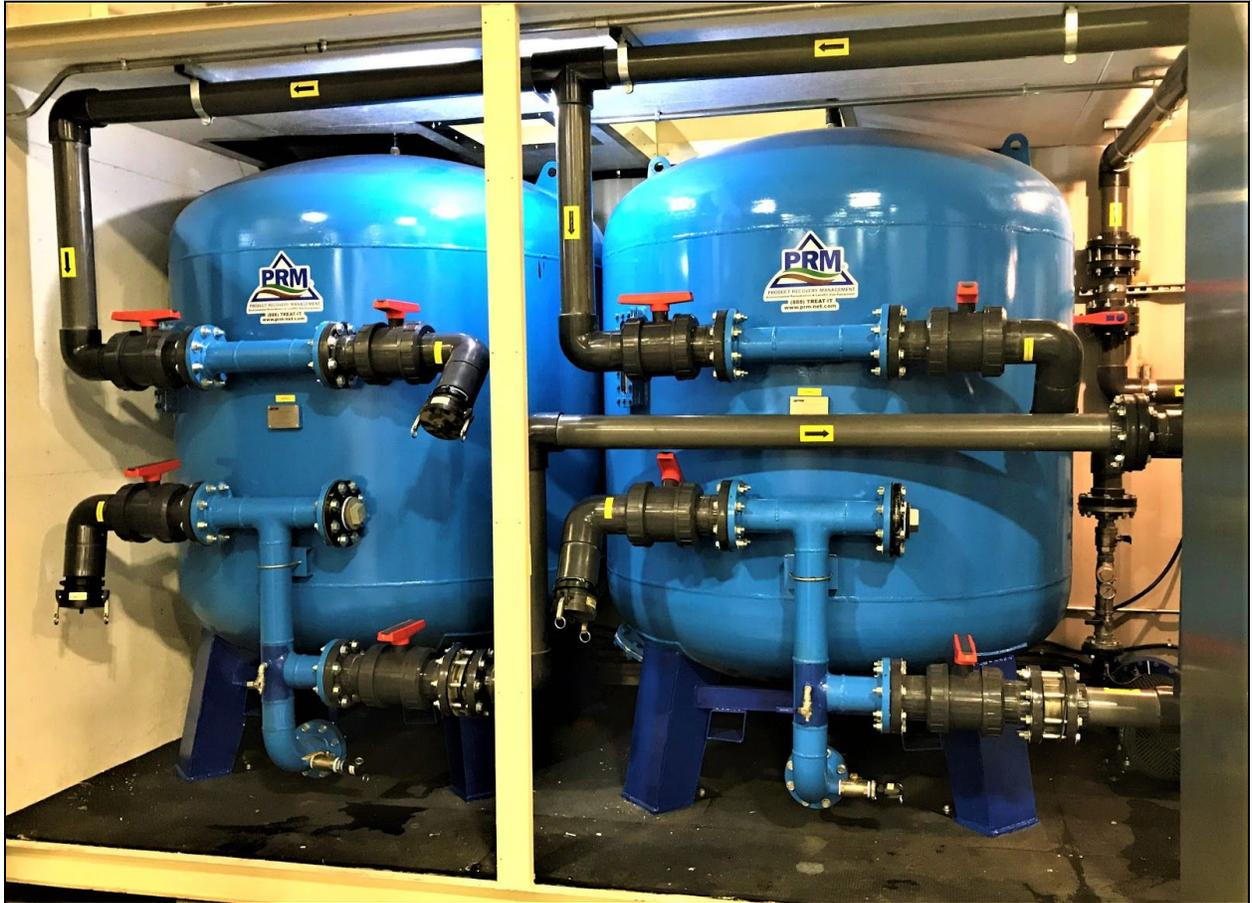
PRM constructed a multi-faceted, comprehensive Groundwater Treatment system. This system is equipped with two inlets, a Gravity Fed inlet and a Vault Pump inlet, dual AMT 3152-98 OWS (Oil Water Separator) Pumps, and two Air Strippers (AST) . Each AST unit has an Ametek EN 909 Series AST Blower. The system is equipped with access ports above the OWS Tank and both Carbon Vessels.
